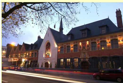
Founded in 1462, l'Hermitage Gantois was a hospice until 1995. It has always welcomed the elderly and the sick of the Lille region, the hospice building being a
